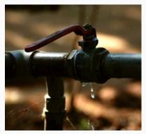
Audible, Visual, and Olfactory detection method (aka: sensory leak detection). In some cases the sensory method is sufficient to meet LDAR requirements – such as MON or 6V Area Source Rule. In most cases it will also start your leak repair clock (5/15).
