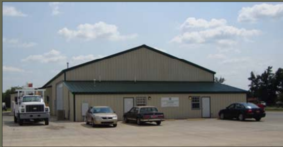
SIP PANEL PLANT
